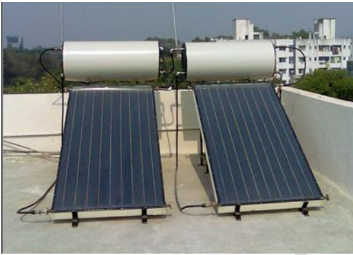
Figure 5.12 Flat plate collector
